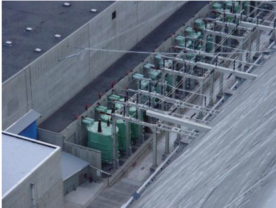
Figure 8.30 Grand coulee hydroelectric dam
