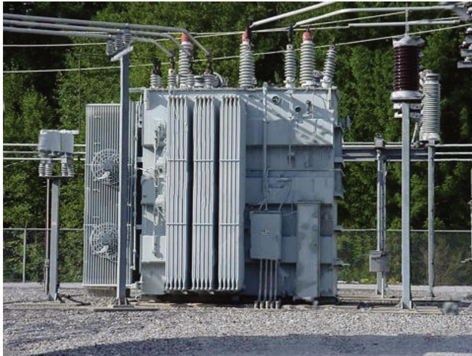
Figure 8.5 Substation transformer.
