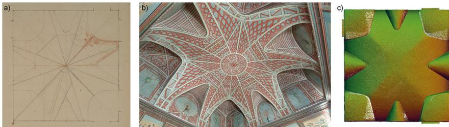
**Fig. 1** Vault of the "Chinese" room in Palazzo Grosso at Riva presso Chieri: **a** Vittone, B. A., study plan for the "Chinese" room vault. ASCRPC, 3\_21/78; **b** photograph of the vault (author's photo); **c** Top view of the point cloud (author's editing)
