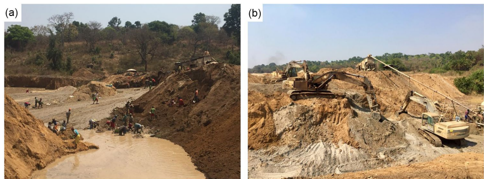
Fig. 3 Artisanal and semi-mechanized mining in the Upper Lom Series a Indigenes panning and recovering gold from the exposed saprolite down to the saprock horizon. b Excavator exposing the saprock layer containing gold for panning
