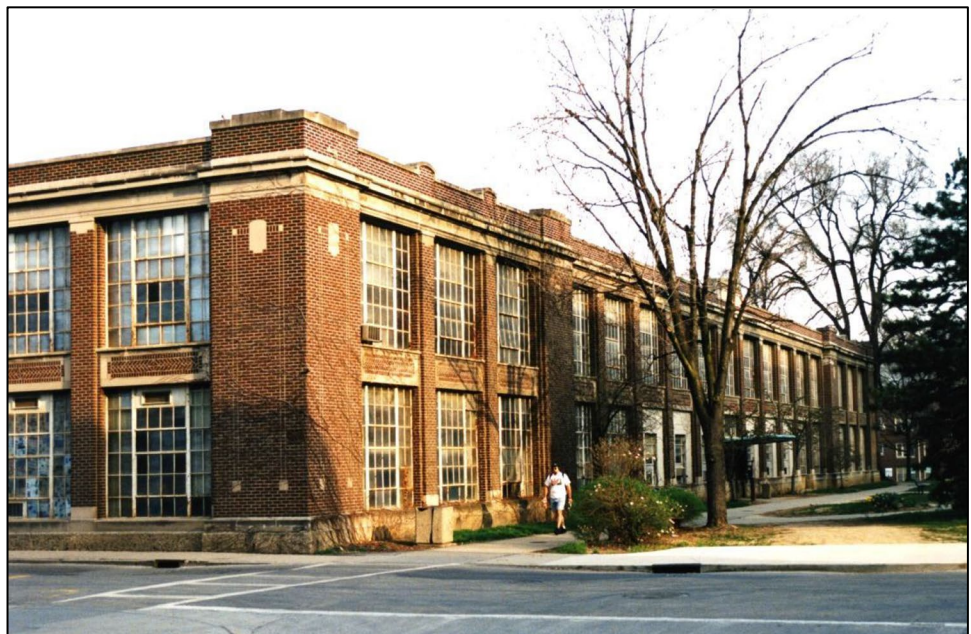
Fig 3 Welding Engineering building on main campus prior to its demolition in 1998
