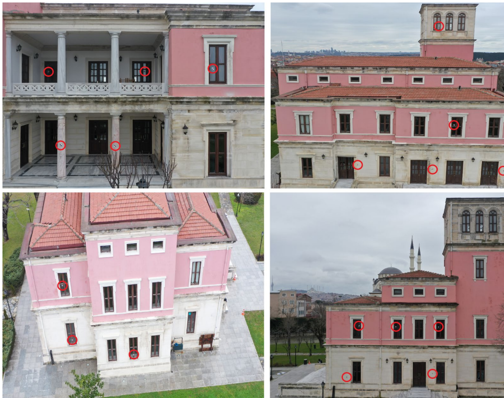
Fig. 4 Building control point locations
