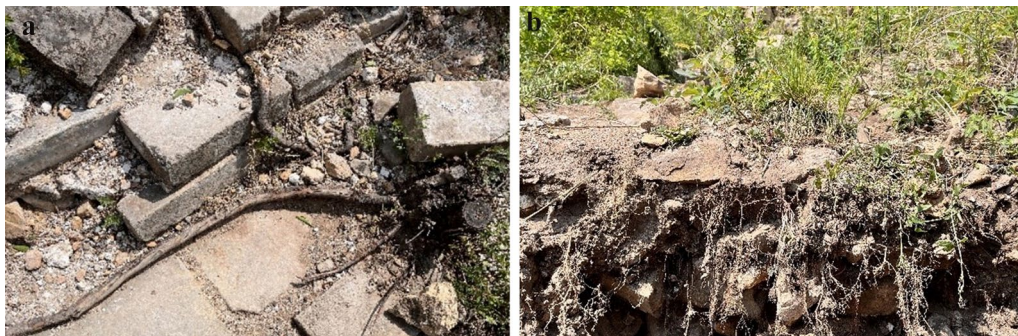
Fig. 4 The status of the Wall-Top Plant root invasion. a Trees and shrubs; b Herbs
