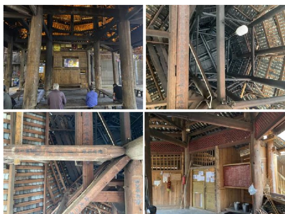
Fig. 2 Internal structure of Dong Drum tower
